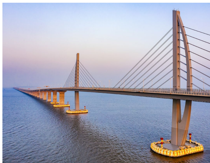
The Hong Kong-Zhuhai-Macau Bridge marked its first anniversary in October 2019.
